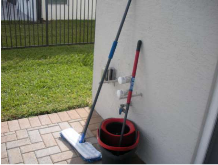
Wall is prepped for outdoor kitchen & Sink
