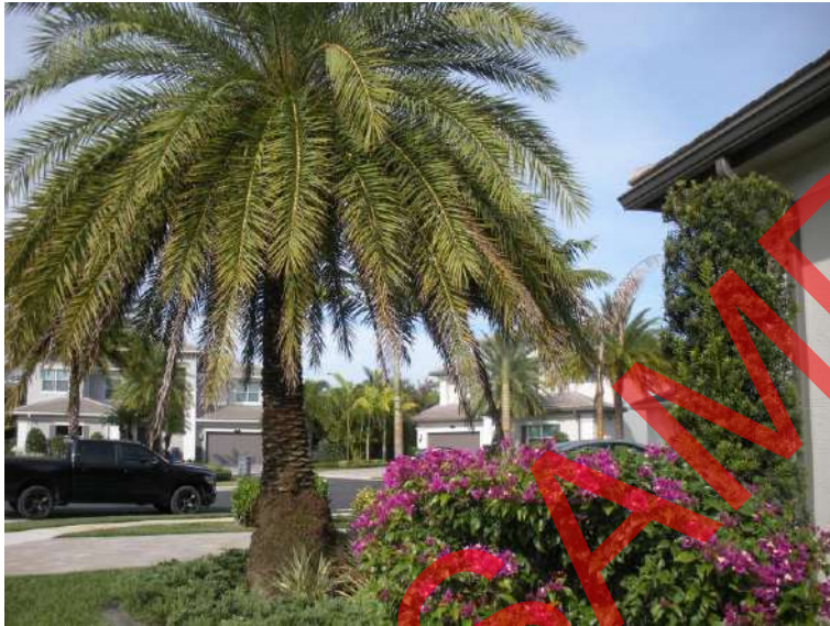
Landscape too close to property is not advised. Standard recommended distance is 2-4 feet away from the structure, to prevent water and insect intrusion.
