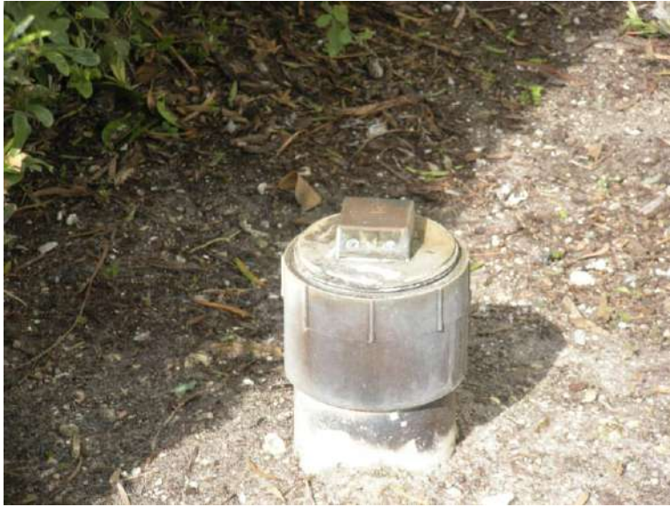
Cleanout pipe is located on the front East side of the property.
