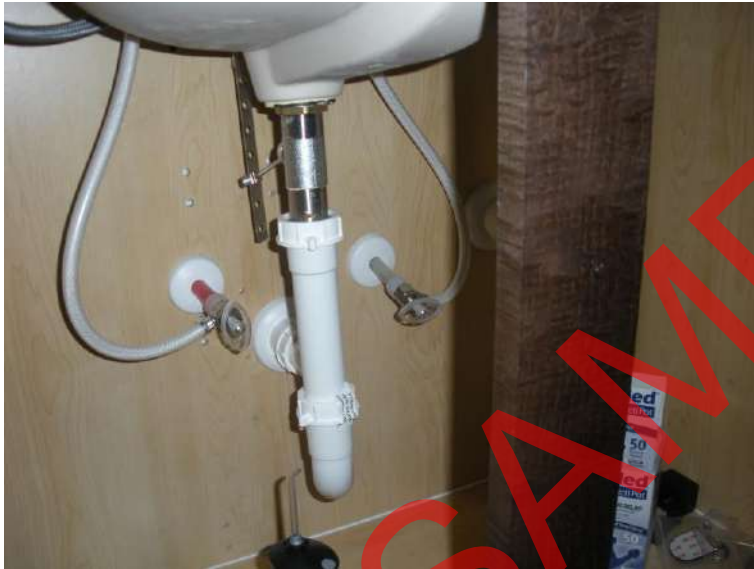
No leaks were present during our inspection
