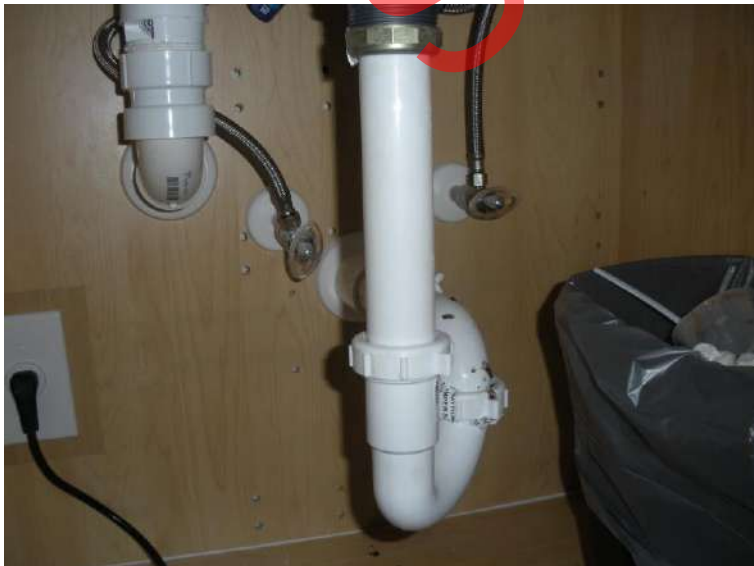
No leaks were present during our inspection
