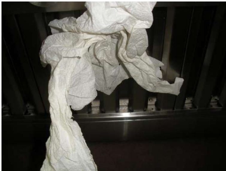
Kitchen vent is operable and pulling air.
